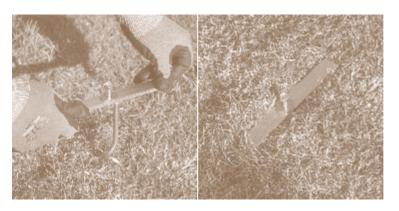
Bolt the screw into the ground
